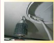
Fasten the box using standard screws for plasterboard at the marks on the box edge
