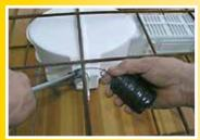
ensure the box to the reinforcing bars, even tying it; pass the cables through the little holes especially made at each side of the boxes.
