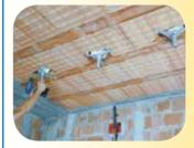
• The special configuration of the application system enables you to achieve a fast and precise positioning of the box at exactly 1 cm. from the brick, leaving enough space for the subsequent plastering.
