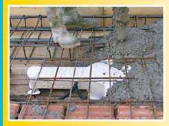
pour the concrete and after that, disarming, we would find the 150mm hole, on the new realised ceiling.
