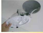
Insert the power supply previously connected
