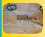
The builder will make the holes in the brick as precisely as possible so as not to complicate later plastering work.
