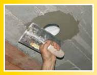
A subsequent shaving with glue tiles or glue for normal plasterboard will allow hiding the remaining grill, leaving space for the perfect hole required.
