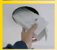
Insert the box into the hole and put it aside
