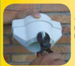
Completely remove the box support which is not necessary in this type of installation.
