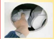
Assemble also the transformer holder
