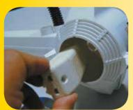
Once the box has been installed, insert the single transformer before installing the spotlight. If the transformer used is of 100w, it is possible to start again from the same box with a short low-voltage line in order to supply another spotlight of 50W installed nearby in a normal TEKPF box.
