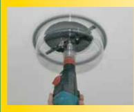
Make the hole after having installed the false ceiling
