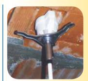
• Using a common extensible pole for paint-rollers, or a builder's sprung perch or, even better, three provisional plugs in the slots, hold the assembly against the unplastered ceiling and keep it steady.
