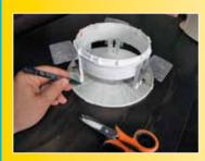
Position the assembly ring nut (frame) over the grill of the light to install, so you can mark its cutting point to contain the ring nut as precisely as possible.
