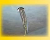
Identify inside the hole made in the false ceiling where the spotlight and the corrugated tubes arranged in advance, which may also have already been strung the wires, will be subsequently installed
