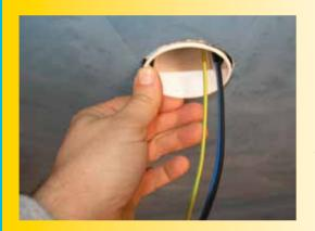
The BOXES TEKPF04 are also suitable for renovations, i.e. in masonry ceilings when already plastered and you have to make the smallest hole possible to avoid damaging the existing ceiling.
