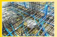
With this accessory the spotlight support box will be raised 5 cm from the surface of the concrete form (recommended height to allow for the concrete to cover the reinforcing bars sufficiently)
