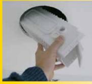
Insert the box into the hole and put it aside
