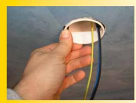
The BOXES TEKPF04 are also suitable for renovations, i.e. in masonry ceilings when already plastered and you have to make the smallest hole possible to avoid damaging the existing ceiling.
