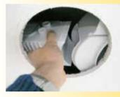
Assemble also the transformer holder
