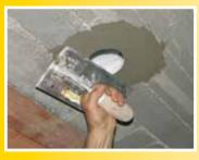
A subsequent shaving with glue tiles or glue for normal plasterboard will allow hiding the remaining grill, leaving space for the perfect hole required.
