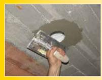
A subsequent shaving with glues tiles or glue for normal plasteboard will allow hiding the remaining grill, leaving space for the perfect hole required. Caution: Do not use lime plaster and cement directly on the grill, make always and firstly the shaving as a support.
