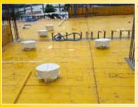
With this accessory the spotlight support box will be raised 5 cm from the surface of the concrete form (recommended height to allow for the concrete to cover the reinforcing bars sufficiently) furthermore it increases the depth of the box.
