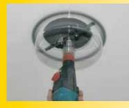
Make the hole after having installed the false ceiling
