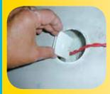
Remember to use the correct cover to separate the lamp space from the transformer space, making sure that the wires are only coming out of the small hole made in the cover for this use.
